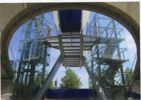
**Above/right** Access to the walkway is by way of a lift or stairs to an assembly platform where 'climbers' are attached to the cable harness system (phs: Buro Happold, Bblur Architecture/Richard Seymour).
