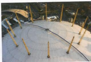
Above The fabric walkway is suspended above the existing structure and runs to its apex with a lanyard cable and handrail running full length. At the top, 53 metres above the ground, is a 12-metre diameter viewing platform. The walkway then extends down to ground level and the exit pavilion on the north side (phs: Bblur/Richard Seymour).
