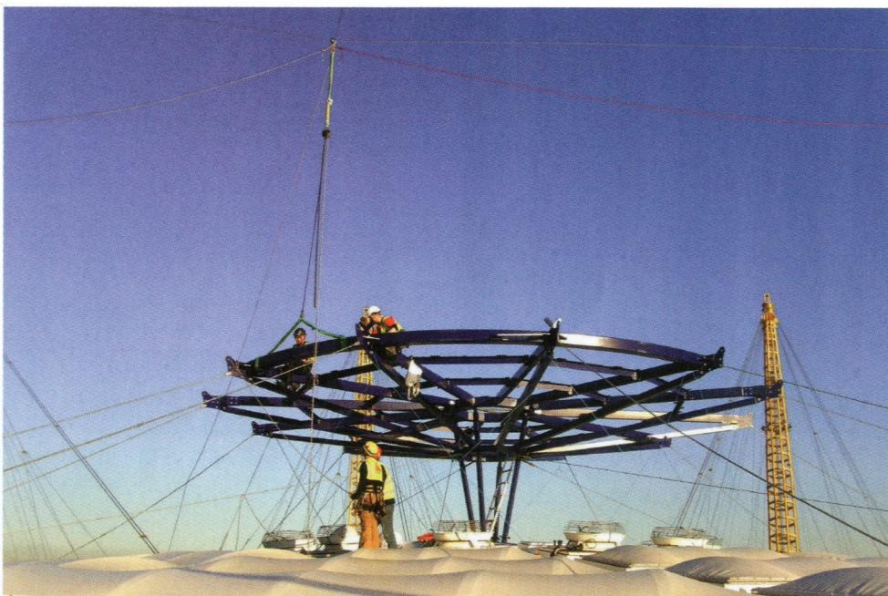
LEFT: Constructing the steel viewing platform. Base Structures ran tension cables between the 100m high masts to allow sky hooks to winch the structure into place.
