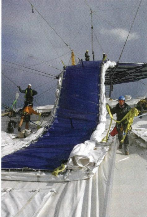
**'Sleds sitting on a temporary fabric PVC 'runway' dragged components up with a Tirfor crank to avoid damaging the O2's roof'**
